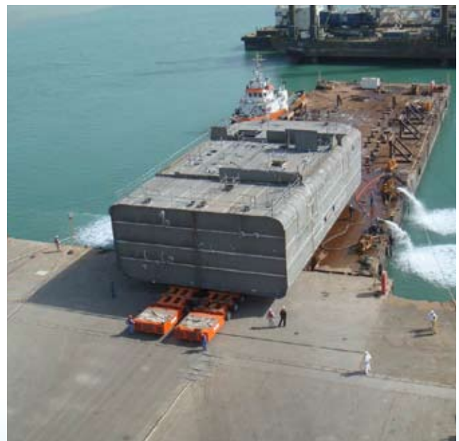
DELBA III Pontoon Section Loadouts/Offloads
