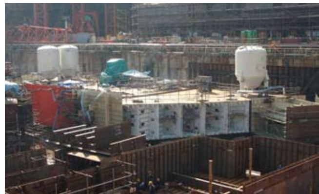
CJ70 Construction - Jurong, 1231A BlockB Drydock
