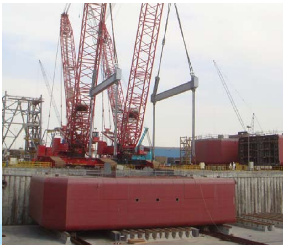
DELBA III Pontoon drydock Installation
