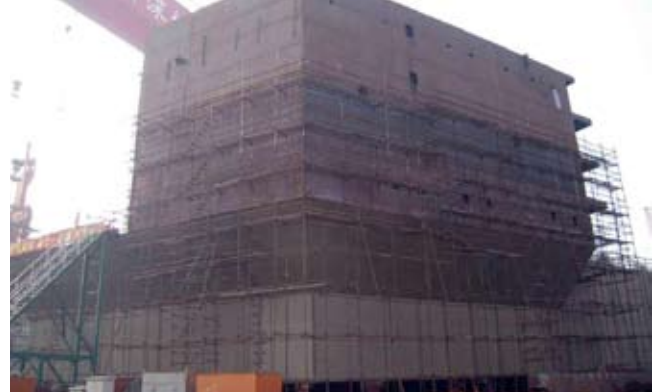
CJ46 construction - COSL936 at CMHI - Hull and accommodation
