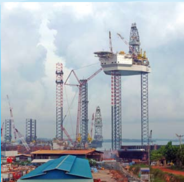
Naga 2 jacking trials at DW/Batam
