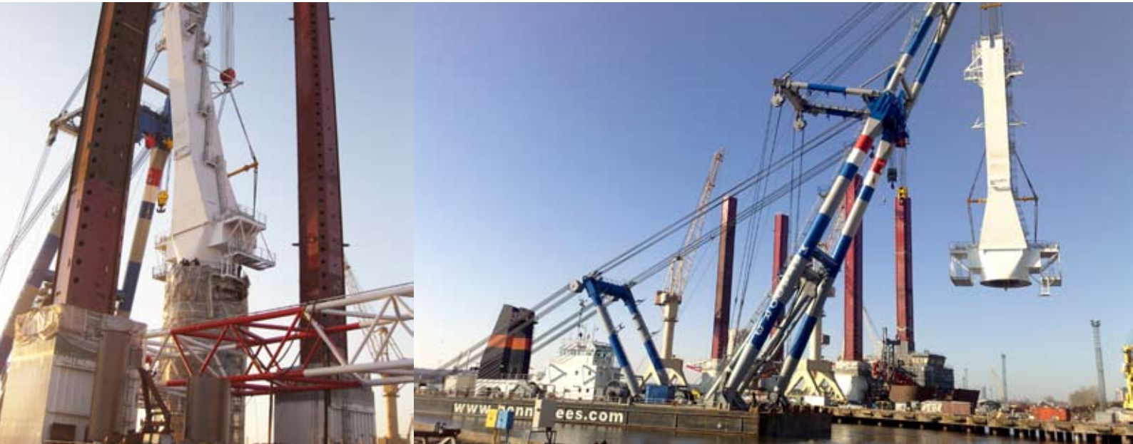
Installation of 500 t crane
