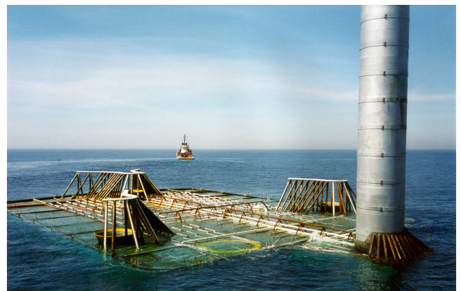
Installation of storage tank
